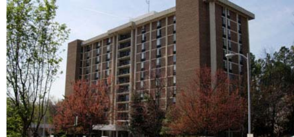
Strawn Hi-Rise Apartments
