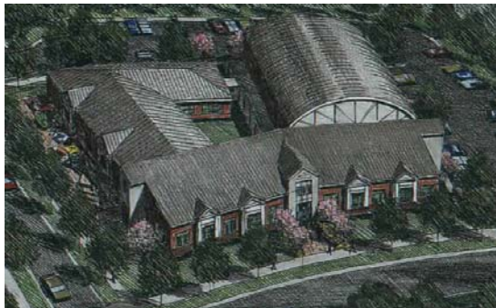
The Park at Oaklawn Community Center
