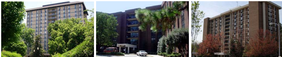
From Left to Right: Edwin Towers, Parktowne Terrace, and Strawn Apartments
